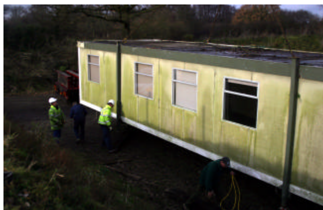
The cabin is lowered into position last December
