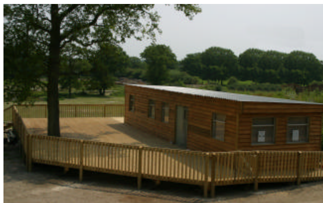
The building nears completion
